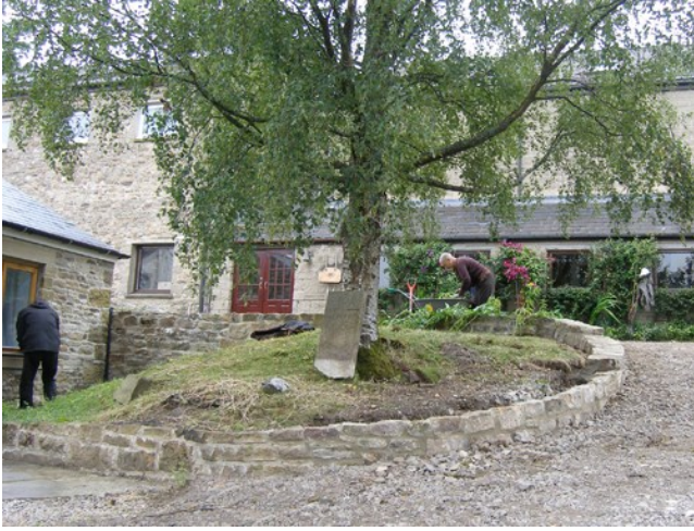
The reconstructed driveway
