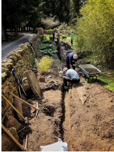
Digging the trench in progress
