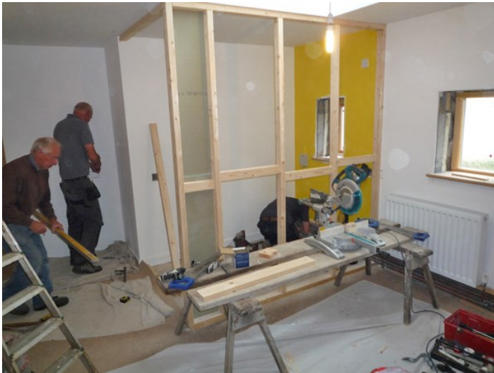
Work in progress on our new bedroom
